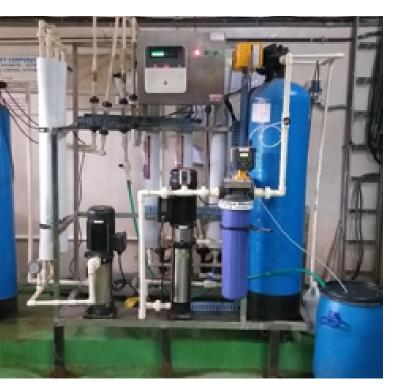
Double pass RO system is comprised of two RO systems. The reject water from 1st pass is further fed to 2nd pass to further recover the water. With this system 57 to 60% water can be recovered unlike single pass RO, which has 30-35% recovery ratio, thus minimising the wastage of water.
