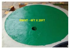
Finished Soak tank covered with a layer of mesh and concrete cap
