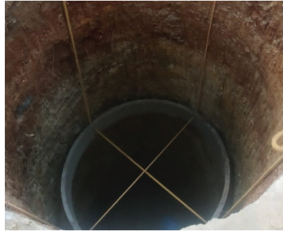
Installation of Concrete rings
