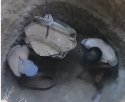
Digging of soak tank
