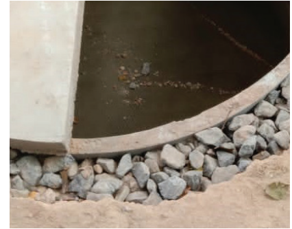
Soak tank surrounding covered with gravels
