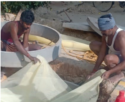
Double layer filter installed for the soak tank
